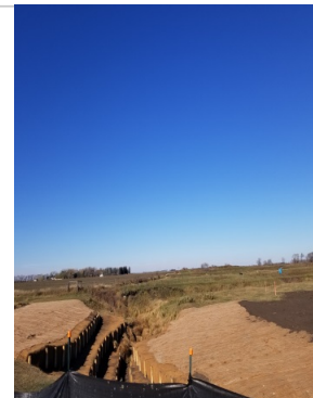
Thornhill Coulee Restoration Jute Matt and Hemp cloth Photo taken North
